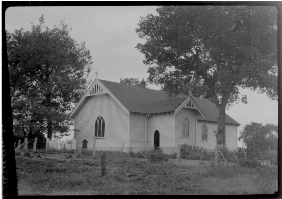
Holy Trinity church, Ngaruawahia, built between 1864–65 by the soldiers of the 12th Regiment.
